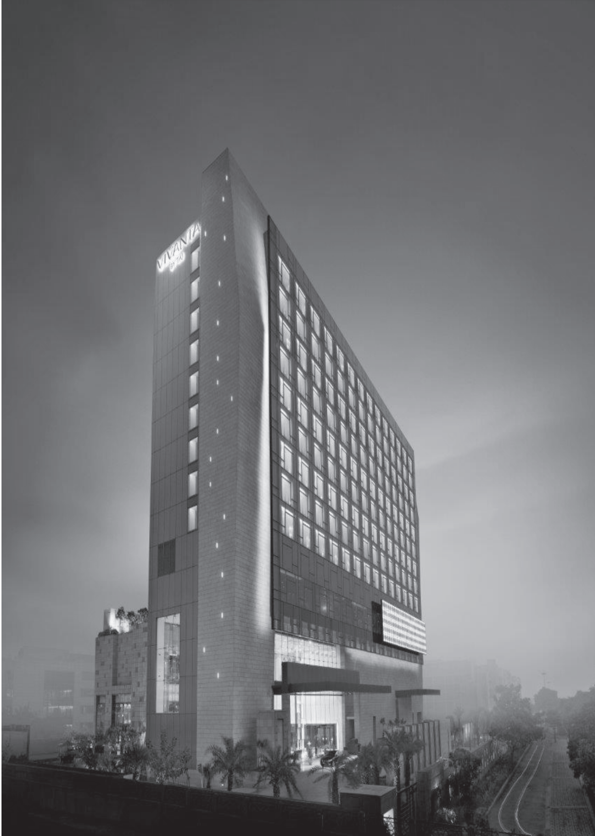
Company's Hotel Project- " VIVANTA BY TAJ - GURGAON, NCR " located at Plot No. 1, Sector 44, Gurgaon, Haryana
