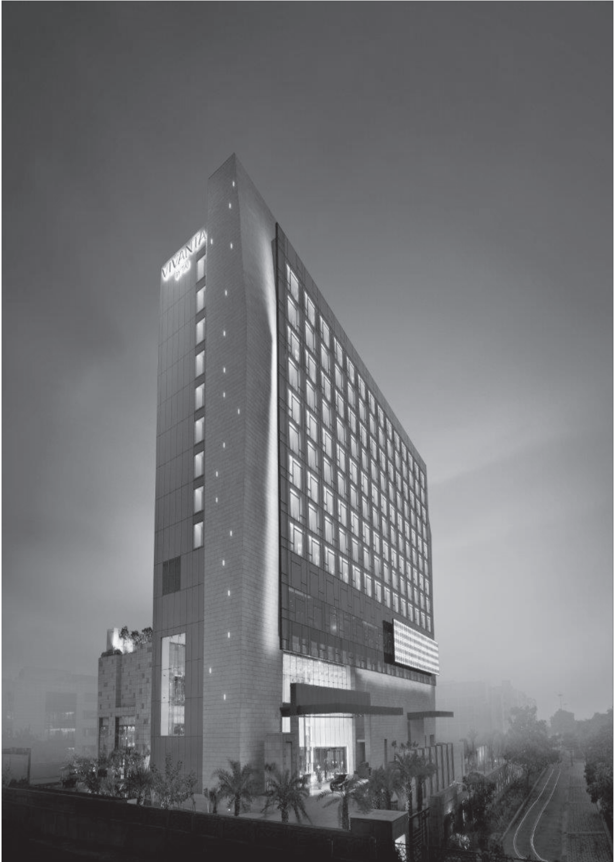
Company's Hotel Project- "VIVANTA BY TAJ - GURGAON, NCR" located at Plot No. 1, Sector 44, Gurgaon, Haryana
