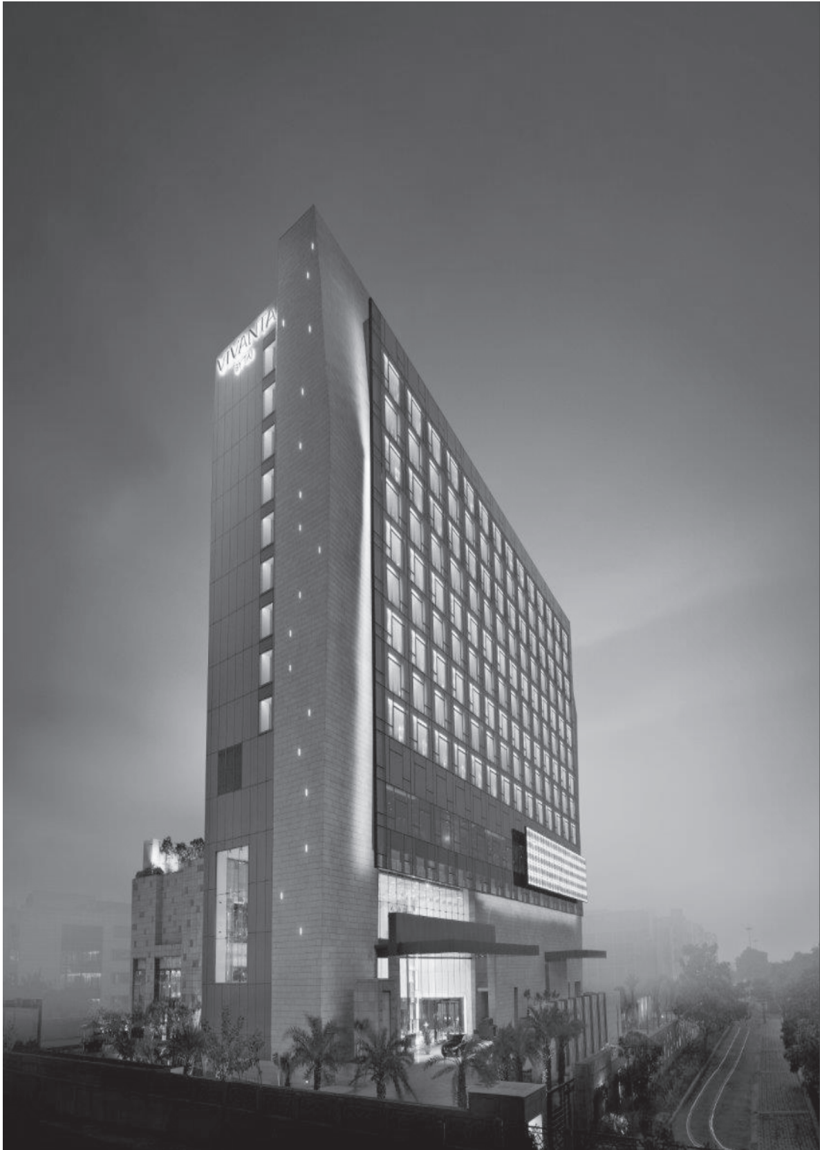
Company's Hotel Project- " VIVANTA BY TAJ - GURGAON, NCR " located at Plot No. 1, Sector 44, Gurugram, Haryana
